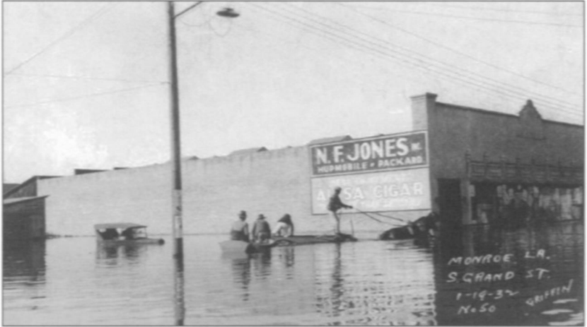
South Grand Street, the main thoroughfare from south Monroe to the downtown area, bore the brunt of the flood damage. Picture from the Ouachita Parish Digital Archive, part of the Special Collections of the Ouachita Parish Public Library, Monroe, Louisiana.
